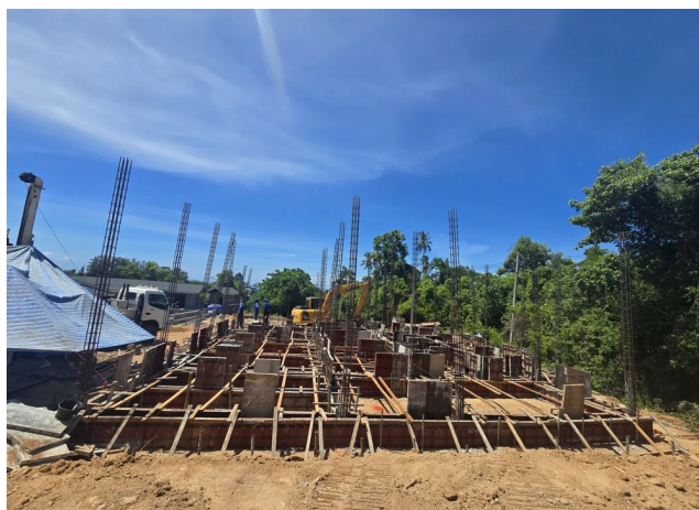
PHOTO 4 Ground beam formwork before the pour
