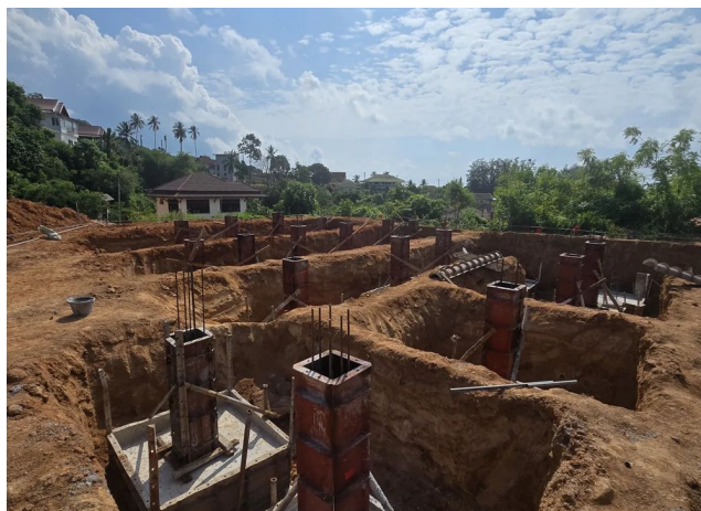
PHOTO 2 Footings poured and column starters
